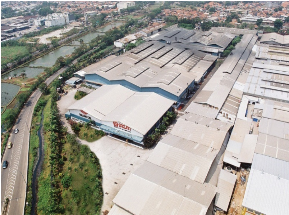
Kapuk Plant (Radiator Facilities)
