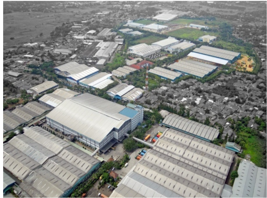
Tangerang Plant (Filter Other Products & Subsidiaries)
